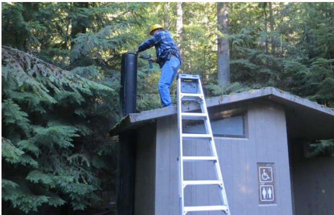
Installing vent caps
