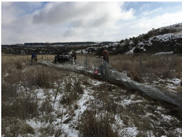
Large enclosure construction
