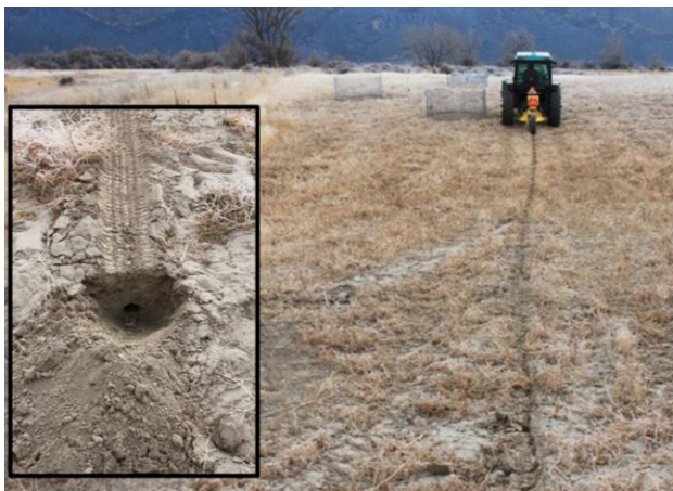
Verminator and finished tunnel
