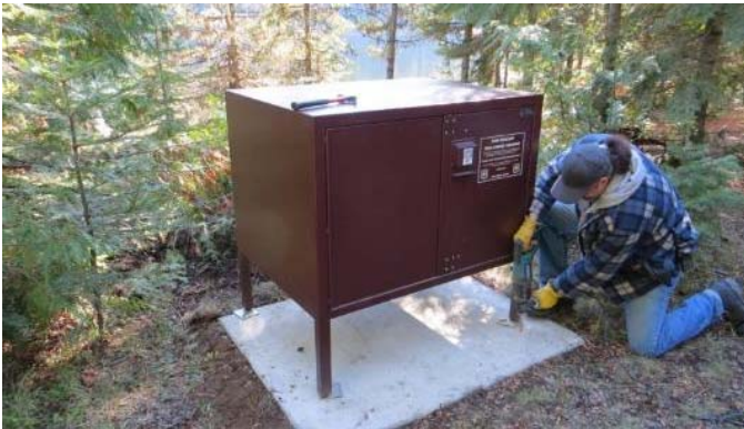
Installing bear-resistant food lockers on the Colville National Forest
