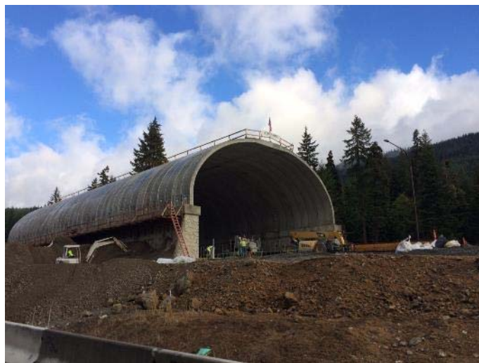
Working on the first arch of the I-90 wildlife overpass
