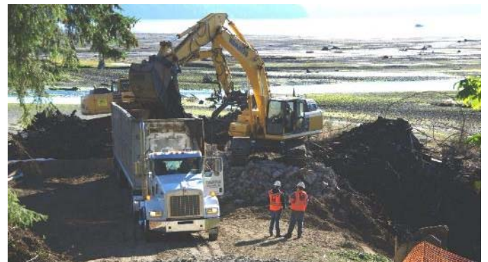
Breaking down the barge to remove it from the estuary
