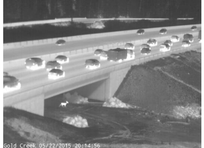
Infrared image of the Gold Creek undercrossing in action
